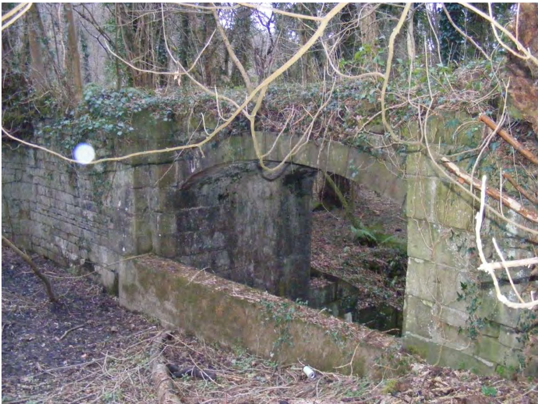
Direction photographer facing: South East
