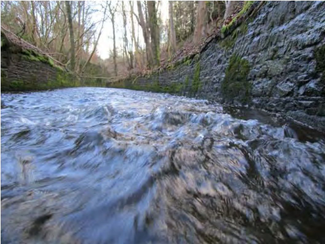
Superb victorian engineering. Stream bed completely flat so water runs from side to side. Direction photographer facing: North
