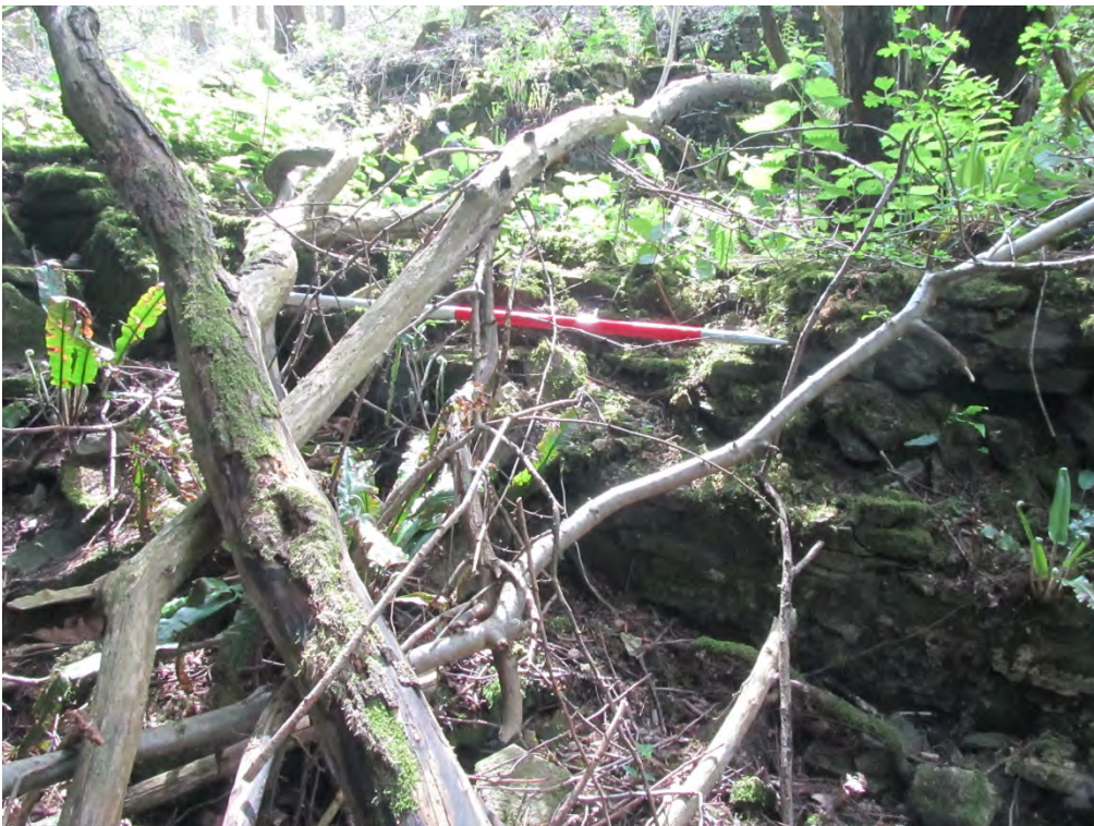
Plate 10: Part of the remains of the east wall of S3 at Tomlin. Photo looking west (Picture Clive Osborne)
