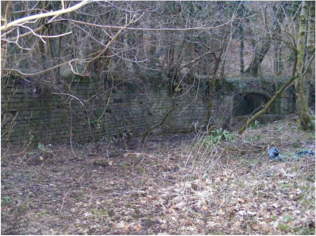
Direction photographer facing: South East
