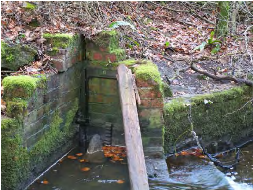
Remains of an old flow control gate. Direction photographer facing: East
